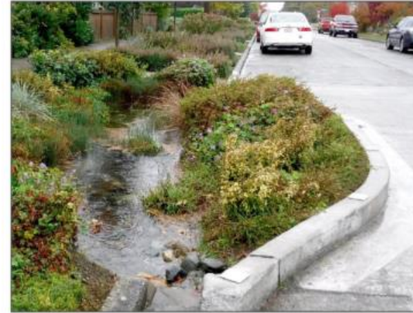
Pictured Above: A curb extension with a bioswale in King County, WA | MIG, 2015. Together, these 93 curb extensions with bioswales function as roadside rain gardens , featuring native and drought-tolerant plants, are estimated to divert six million gallons of stormwater annually from entering the combined sewer overflow.
