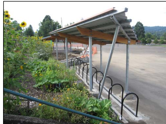
Camas Ridge Covered Bicycle Parking with Rainwater Catchment System. Photo by Shane MacRhodes.
