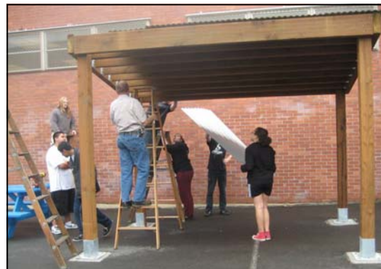
Volunteers Construct Portland Public Schools Bike Shelter. Photo by Anne Laufe with the Oregonian.
