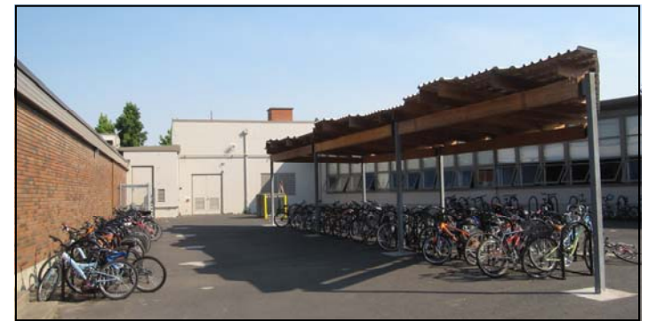
Upgraded Covered Bicycle Parking at Roosevelt Middle School. Collaboration Project with University of Oregon
