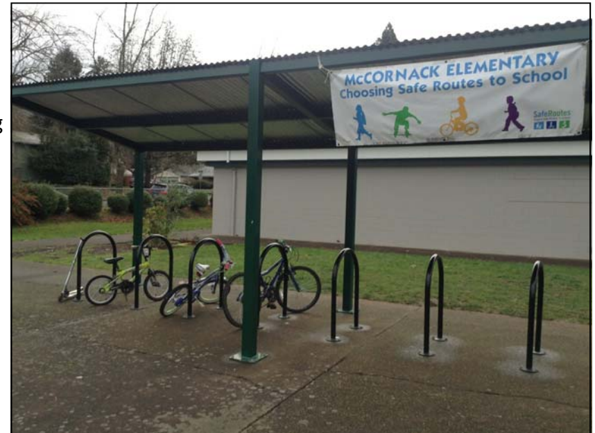
Covered Bicycle Parking at McCornack Elementary School. Photo by Shane MacRhodes.
